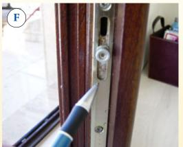
simply a small gap between the door handle and the faceplate, which allowed water to enter and run down through the three-point locking mechanism. Note the rust spot on the hardware (F) where the water came in. We recommended adding a rubber washer between the handle and the plate — an inexpensive fix, considering how much money had been invested in trying to solve the problem.
