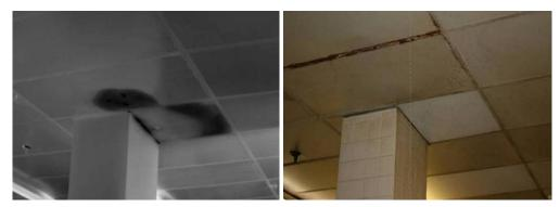
Figure 5 – Uninsulated column passing from cool area into the warm, moist interstitial space, causing condensation on the column, which then drips onto the ceiling tiles.
