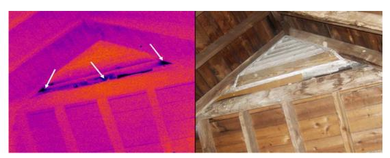
Figure 1 – Water entering the attic of a large church at the gable end vent.
